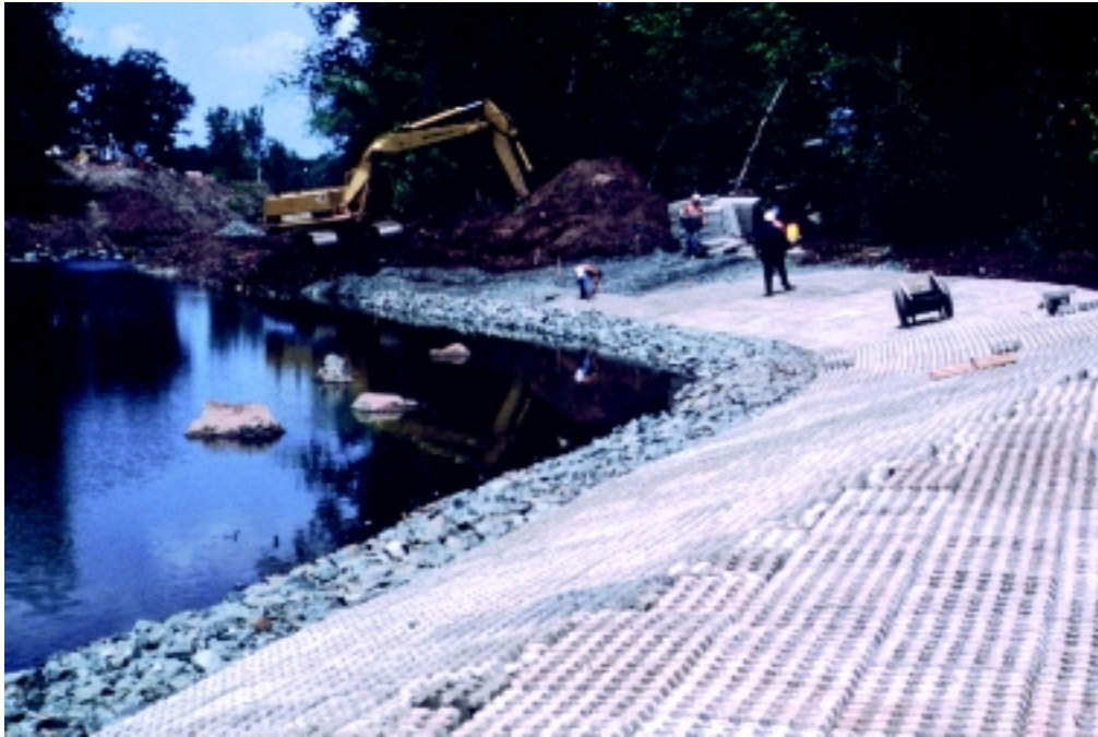
Figure 16-35a Concrete cellular block system before backfilling
