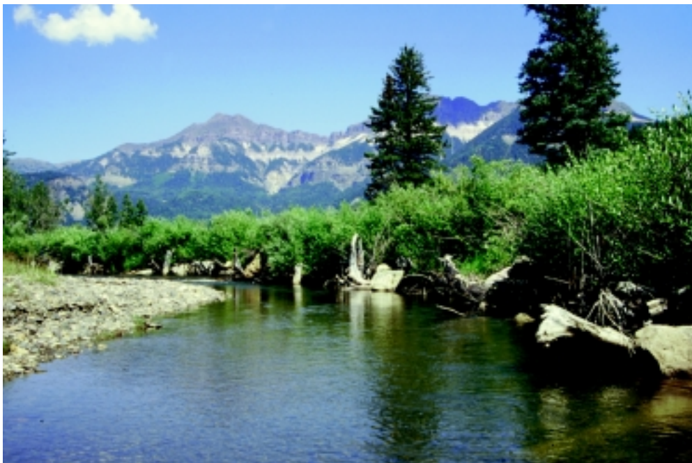
Figure 16-23 Rootwad, boulder, and willow transplant revetment system, Weminuche River, CO (Rosgen, Wildland hydrology)
