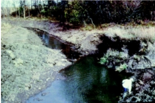
Figure 16-15a Pre-construction streambank conditions
