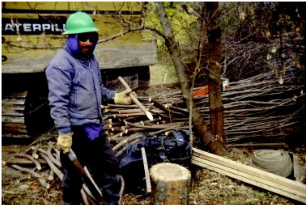
Figure 16-5 Prepared live stake (Robbin B. Sotir & Associates photo)
