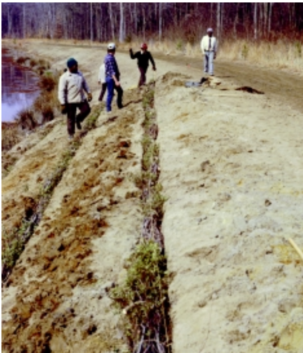
Figure 16-9a Placing live fascines (Robbin B. Sotir & Associates photo)
