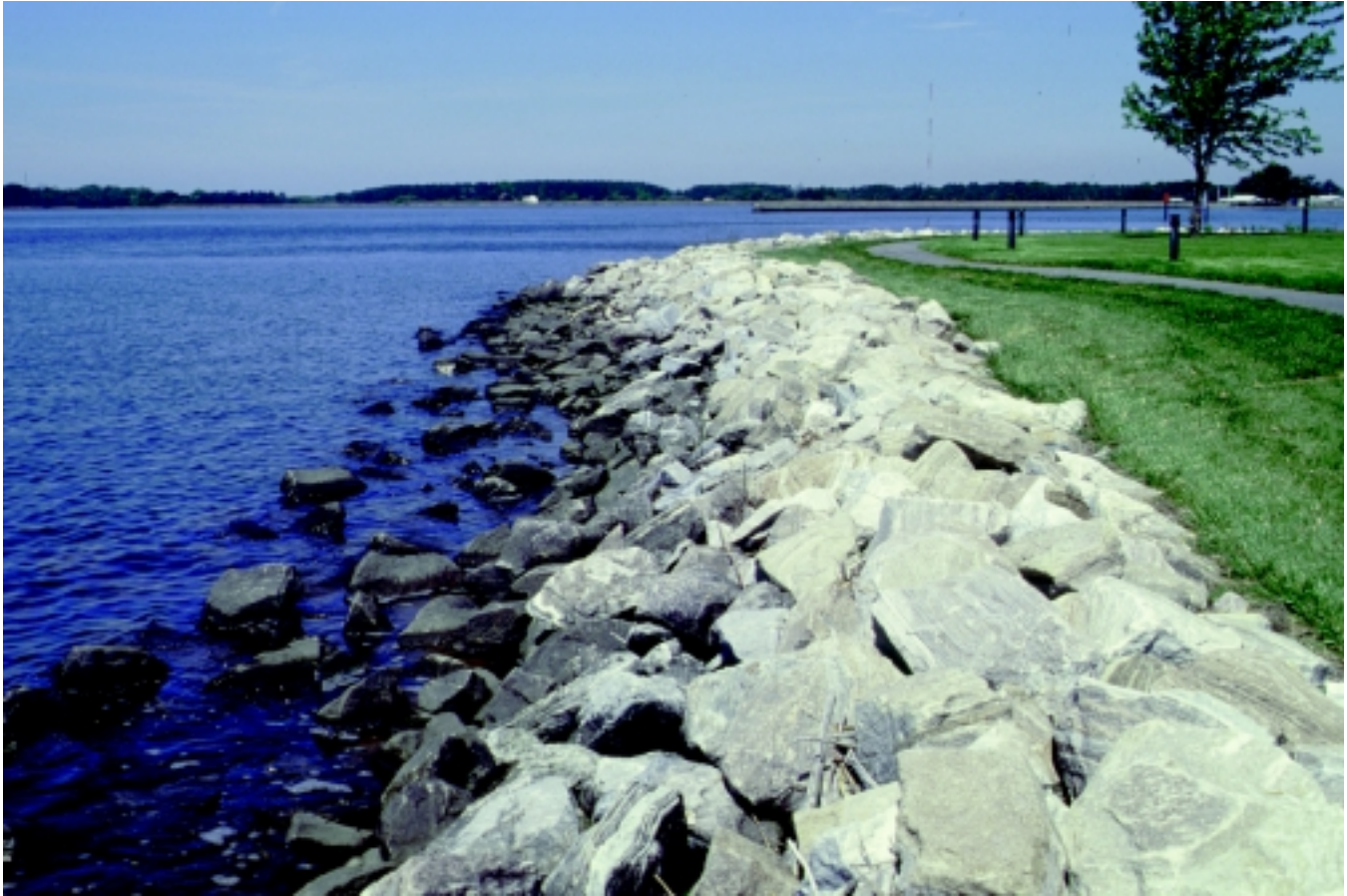
Figure 16-51 Rock riprap revetment
