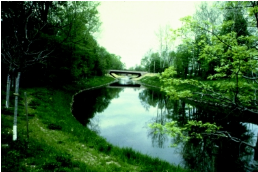
Figure 16-35b Concrete cellular block system several years after installation
