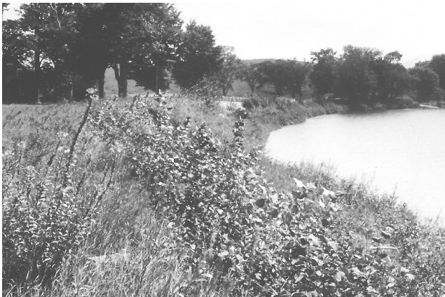
Figure 16-3c Three years after installation of soil bioengineering practices, 1941
