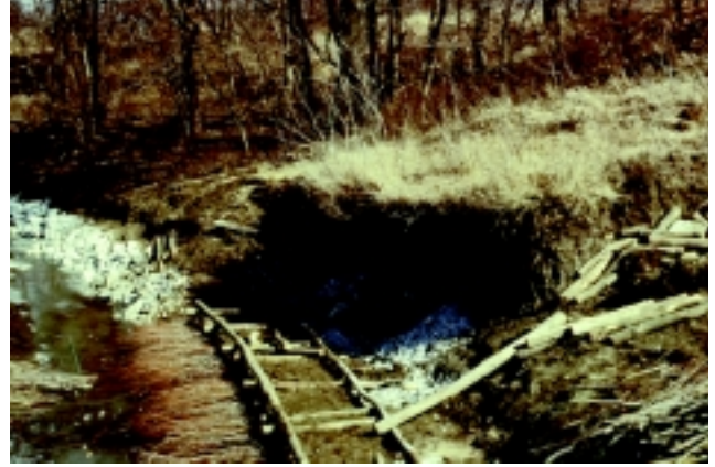
Figure 16-15b A live cribwall during installation
