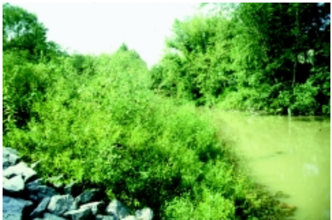
Figure 16-19d Brushmattress system 2 years after installation (Robbin B. Sotir & Associates photo)
