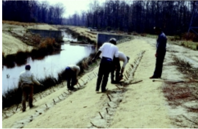
Figure 16-9b Installing live stakes in live fascine system (Robbin B. Sotir & Associates photo)
