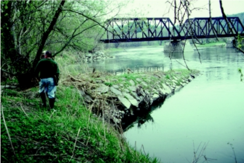
Figure 16-39a Stream jetty placed to protect railroad bridge
