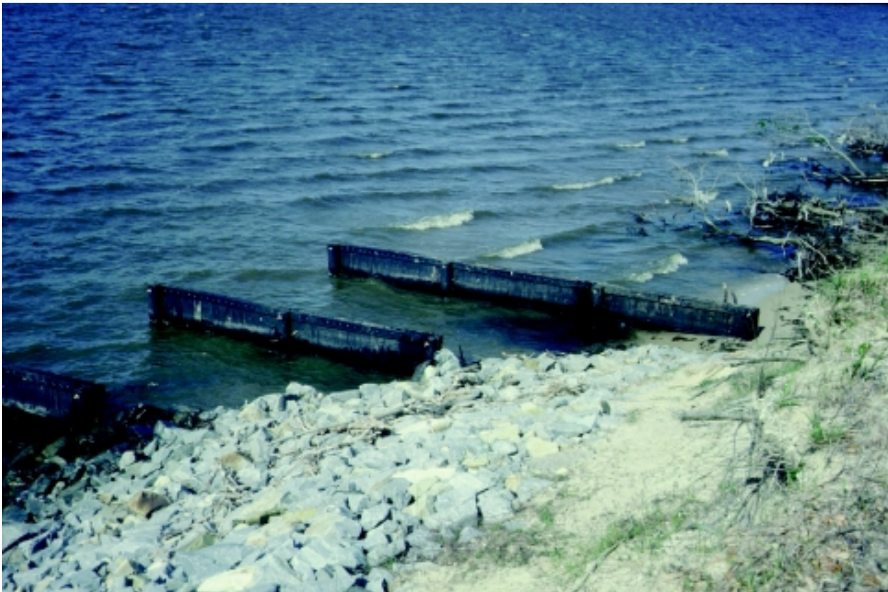
Figure 16-45 Timber groin system
