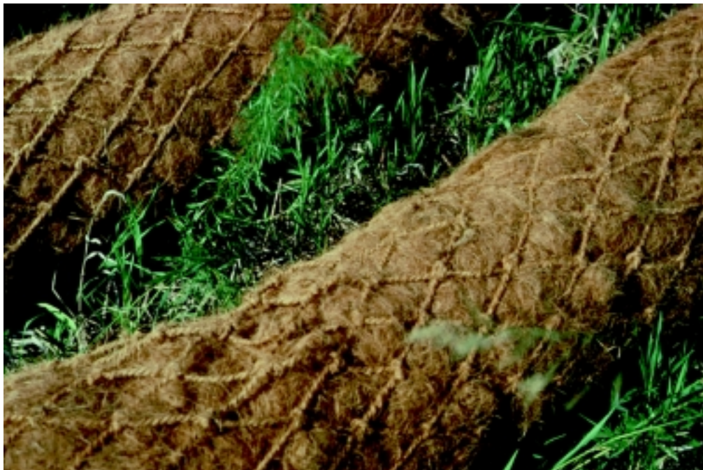
Figure 16-37a Coconut fiber roll
