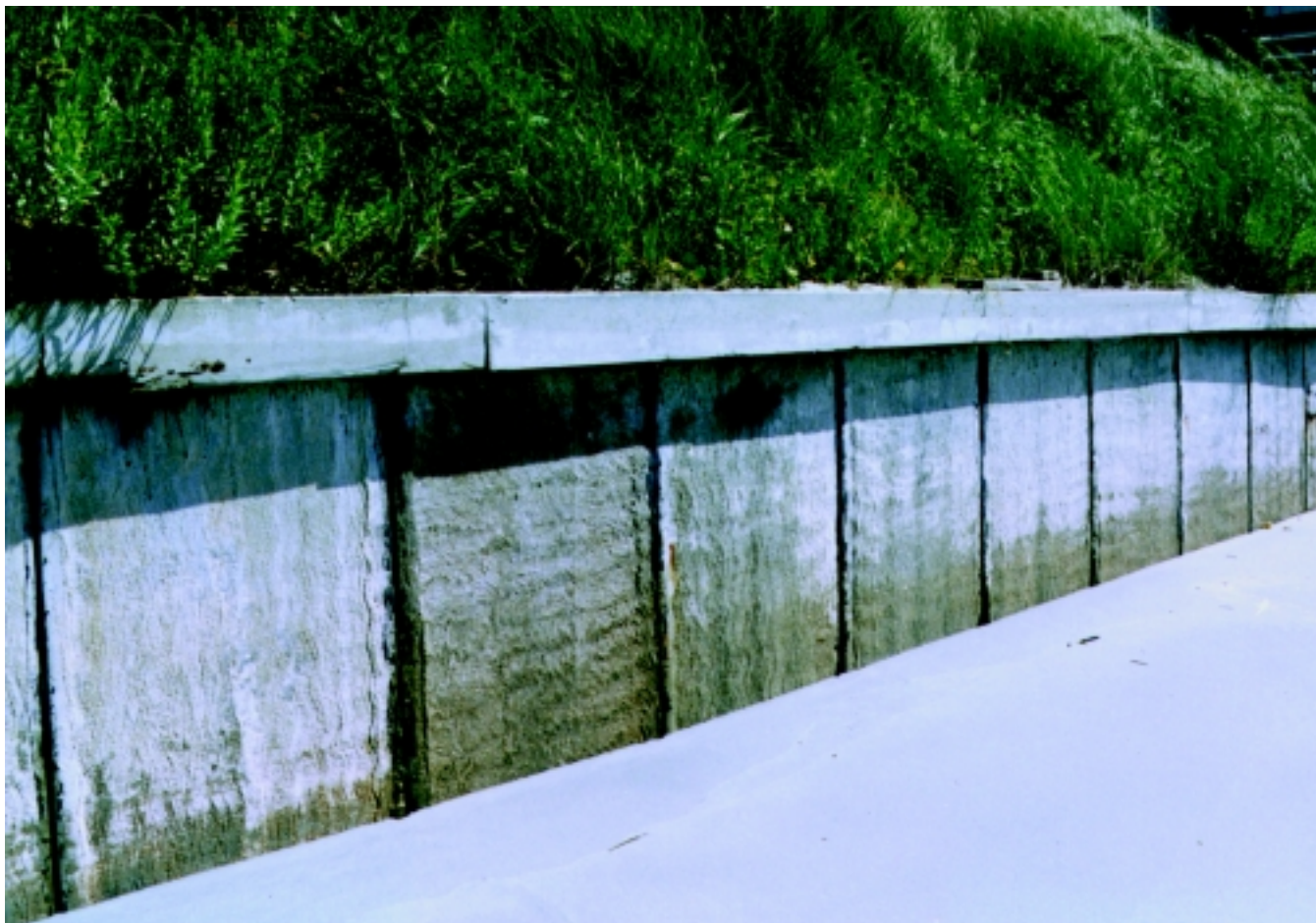
Figure 16-49 Concrete bulkhead system
