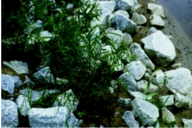
Figure 16-17a Live stake tamped into rock joints (joint planting) (Robbin B. Sotir & Associates photo)
