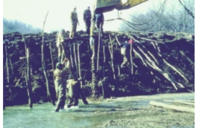
Figure 16-25b Installing dormant posts (Don Roseboom photo)
