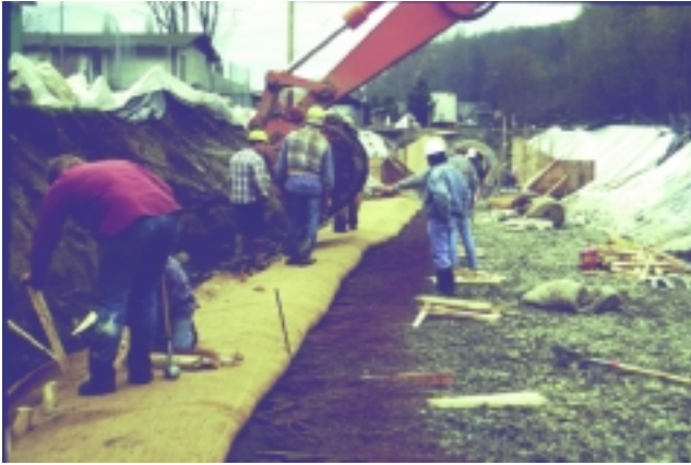
Figure 16-13a A vegetated geogrid during installation (Robbin B. Sotir & Associates photo)
