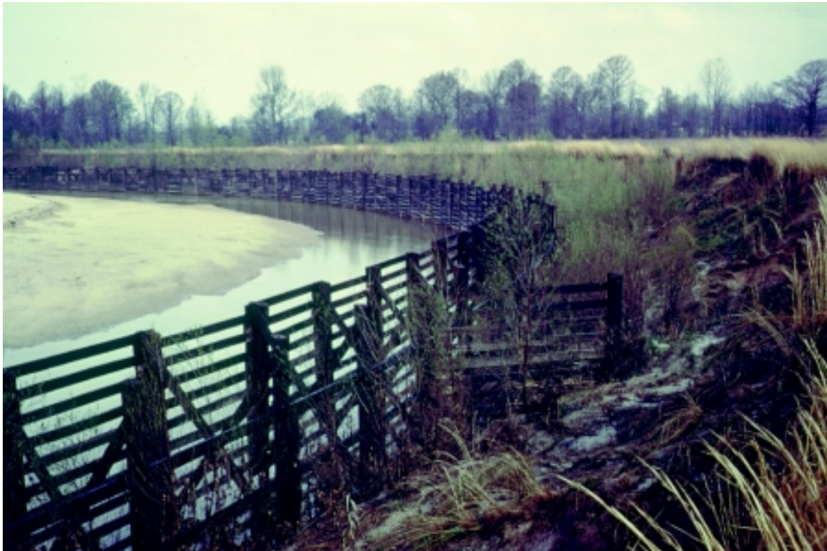
Figure 16-28 Slotted board fence system
