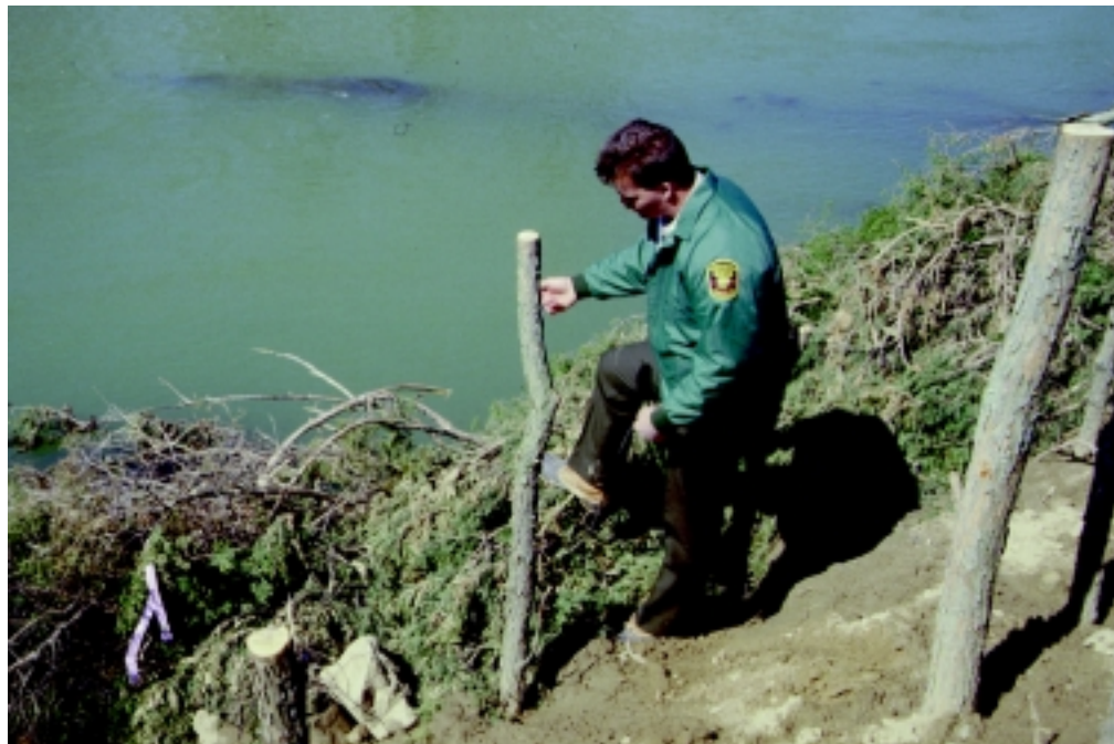
Figure 16-21a Tree revetment system with dormant posts
