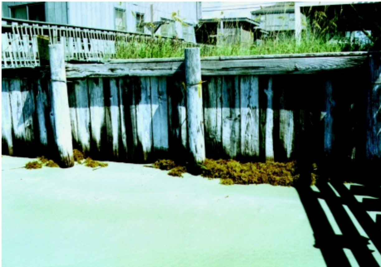
Figure 16-46 Timber bulkhead system
