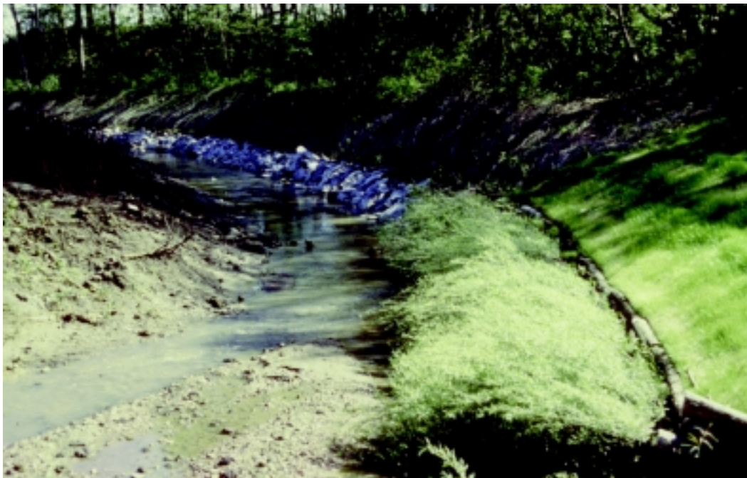
Figure 16-15c An established live cribwall system
