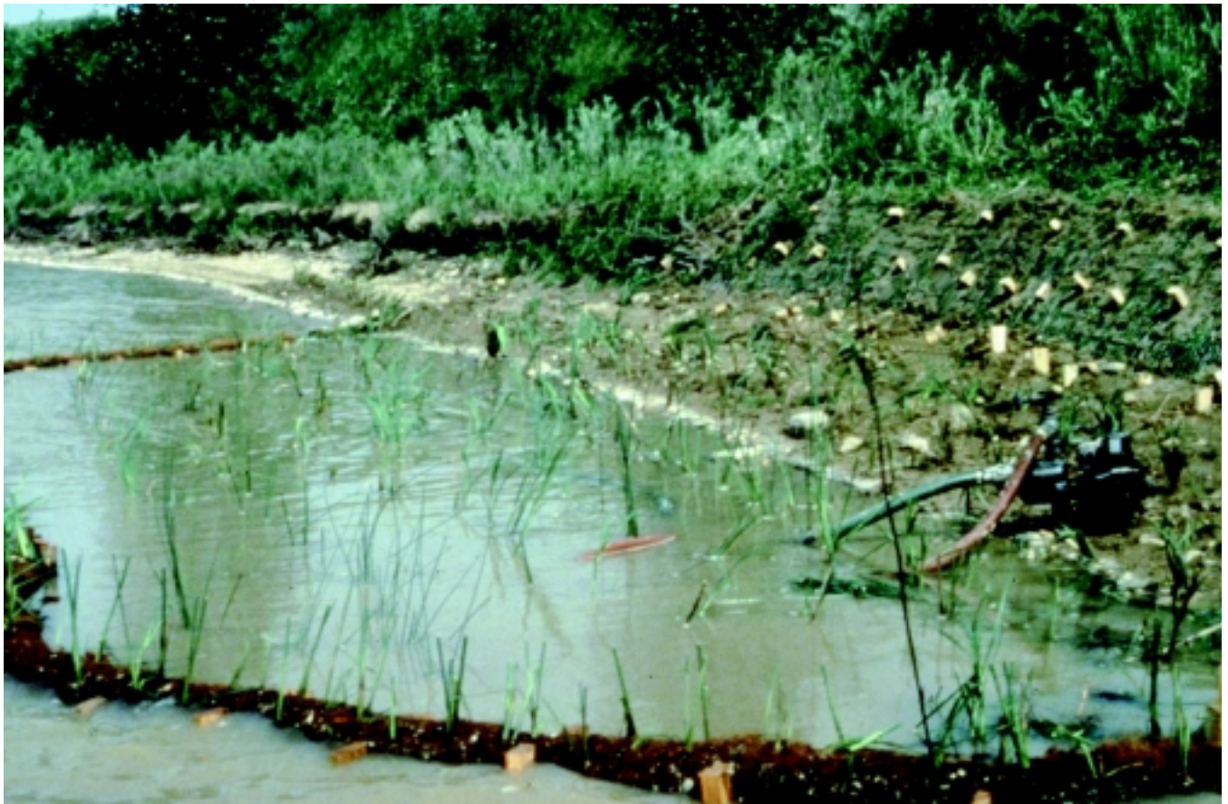
Figure 16–57 Coconut fiber roll system
